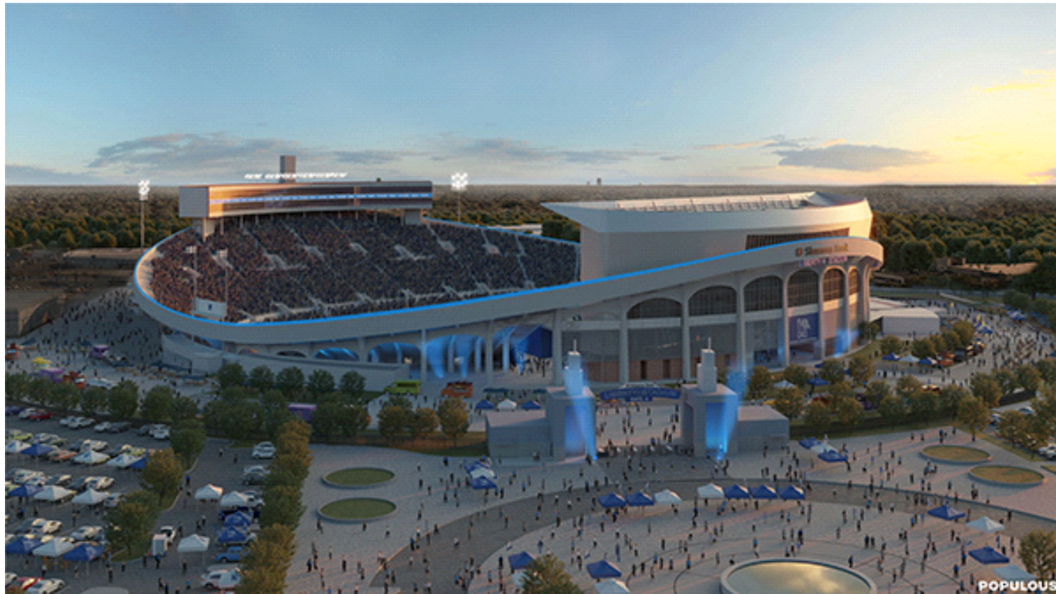
Phase 2 of Simmons Bank Liberty Stadium is underway to provide fans with great game day experience. Above is a rendition on how the new stadium will look. Behold the beauty of a winning season! (Photo/Courtesy: UofM Athletics)
